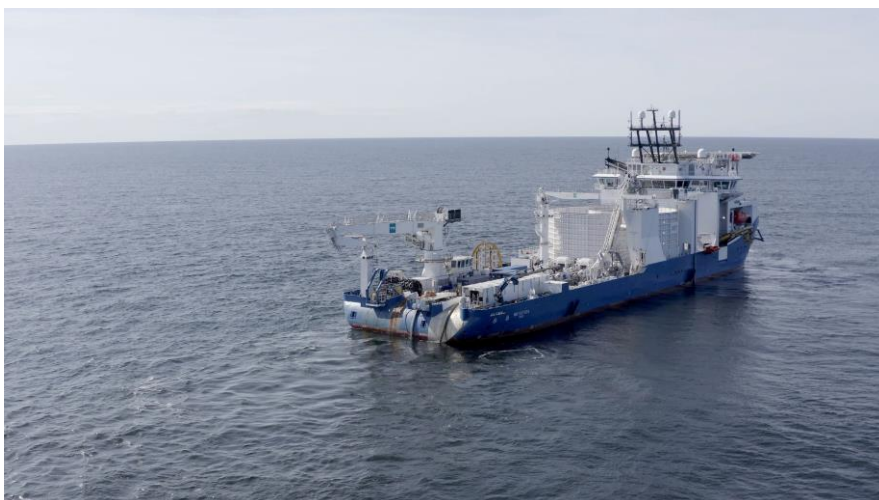
The submarine cables for NordLink are laid from a ship.
